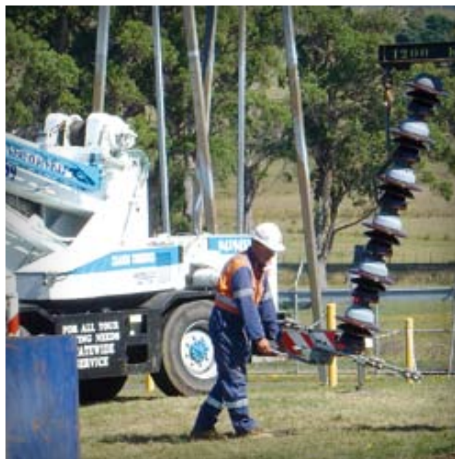
An old insulator is removed at Sheffield Substation
