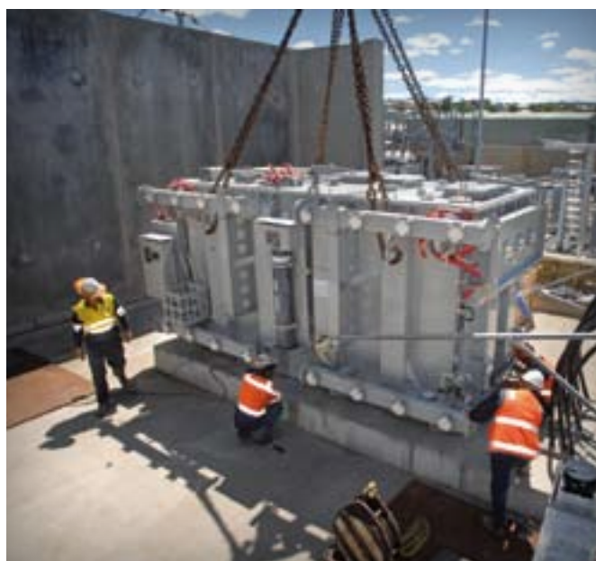
A new transformer being installed at Mowbray Substation, Launceston
